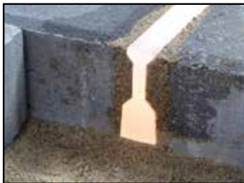
side view of Pavelux® installed
